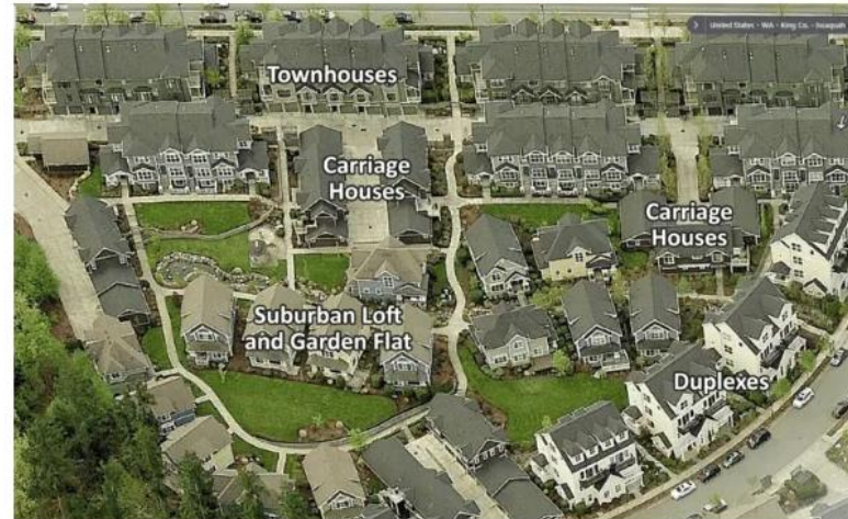
RELATIVELY NEW MIXED-HOUSING-TYPE SUBDIVISION, ALSO WITHIN THE MASTER-PLANNED ISSAQUAH HIGHLANDS DEVELOPMENT IN ISSAQUAH.
