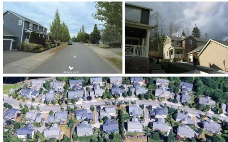
RELATIVELY NEW SINGLE-FAMILY SUBDIVISION WITHIN THE MASTER-PLANNED SNOQUALMIE RIDGE DEVELOPMENT IN SNOQUALMIE.
